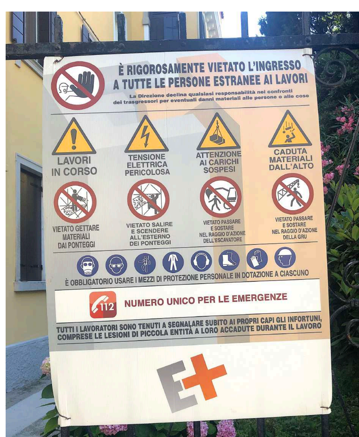
Fig 9. Warning Sign at Construction Site, Fondamente Santa Marta (28.6.23).
